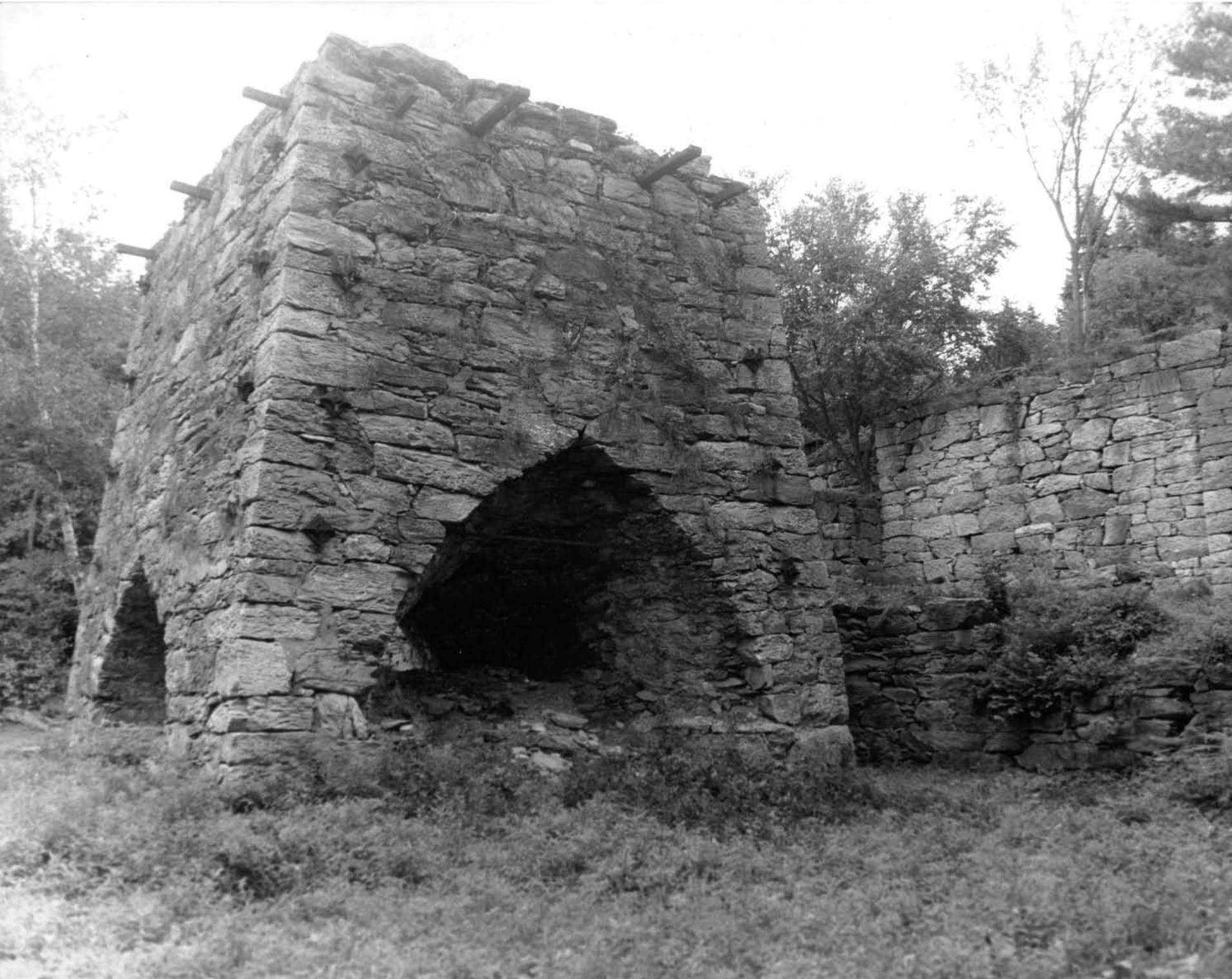
14. Blast Furnace, looking northeast (Photographer: Matthew A. Kierstead, August 1997)
