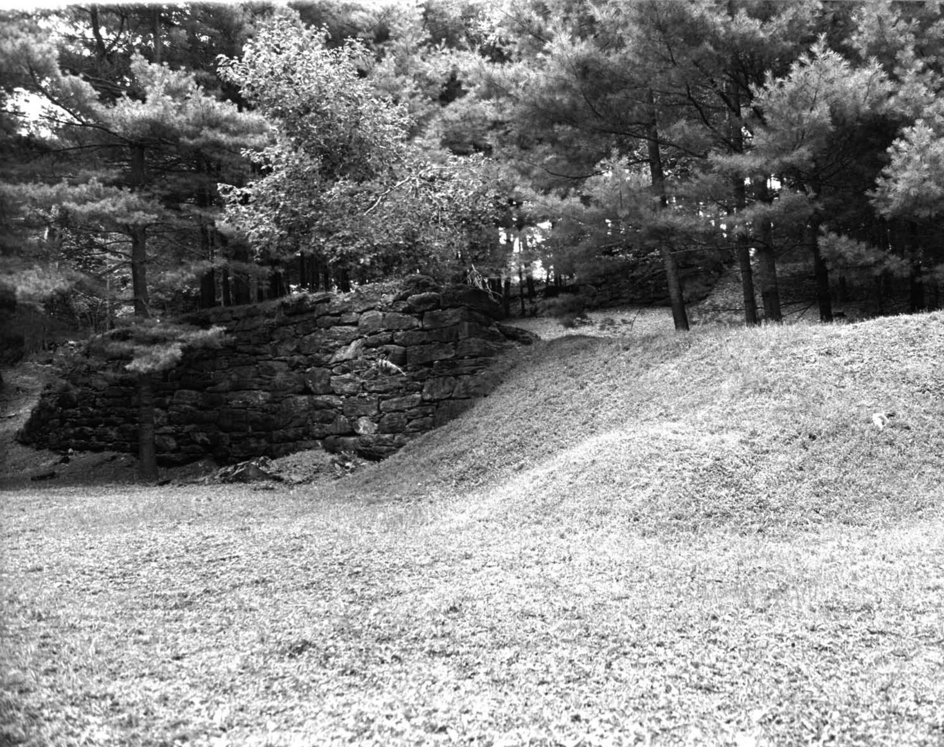
6. Cone Mine Ore Crusher and Washer House Upper and Lower Foundations, looking northeast (Photographer: Matthew A. Kierstead, August 1997)
