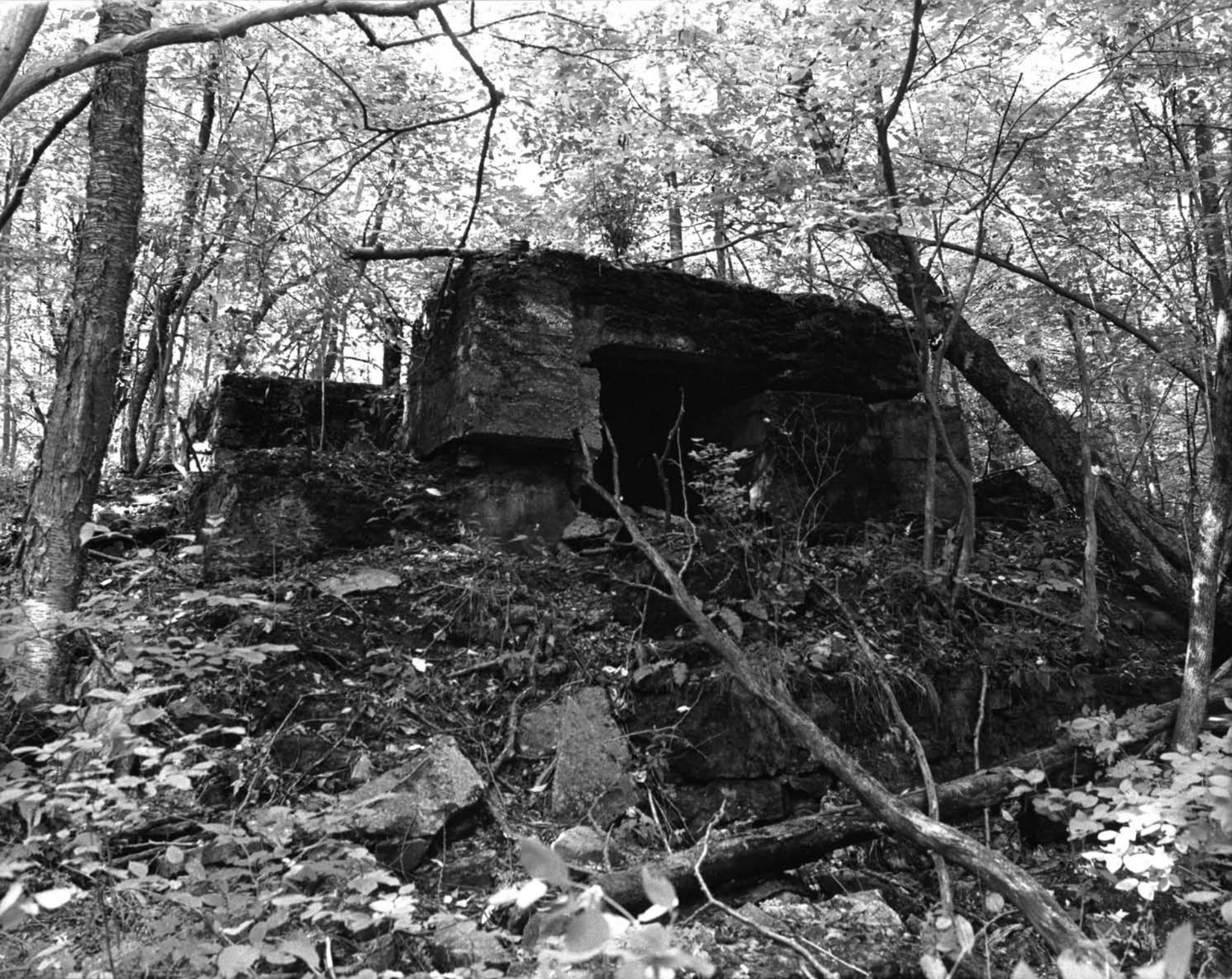
7. Klondike Mine Ore Crusher/Washer House Foundation, looking north (Photographer: Matthew A. Kierstead, August 1997)
