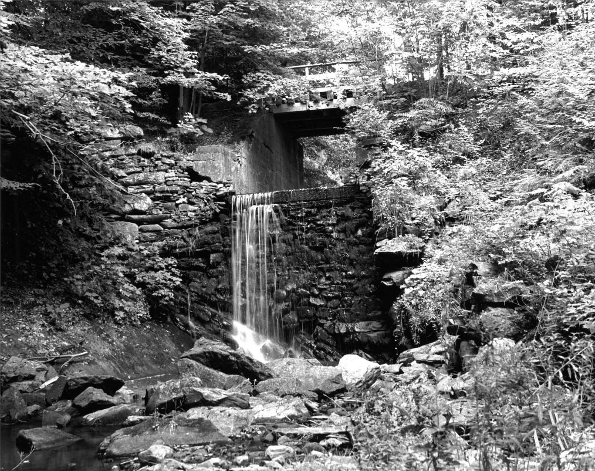
12. Furnace Pond Main Dam, Bridge, and Spillway, looking north (Photographer: Matthew A. Kierstead, August 1997)
