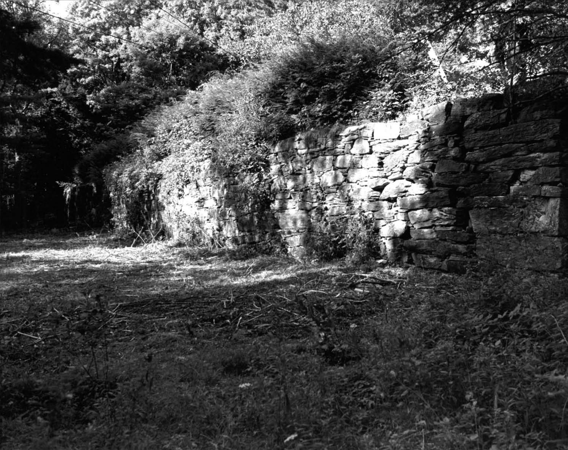
13. Charcoal Shed Foundation, looking northeast (Photographer: Matthew A. Kierstead, August 1997)
